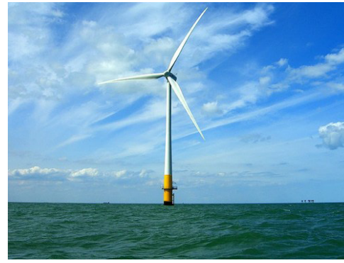
Offshore Wind Turbine
