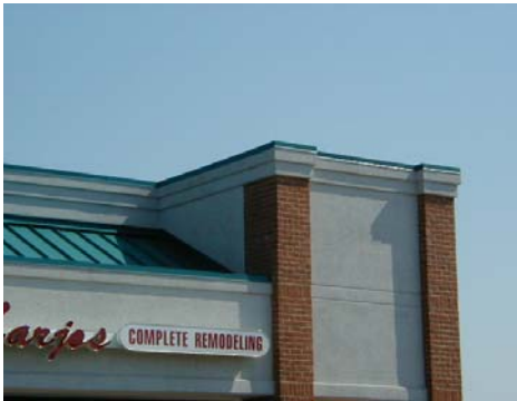
Combination of brick, texture concrete masonry.
