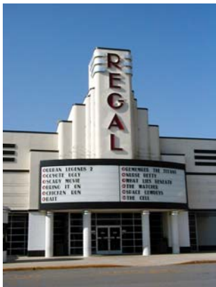
Entryway design using Recesses, Projections, Overhangs and Architectural details which are integrated into the building structure and design.
