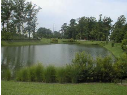
A natural landscaped storm water management facility.
