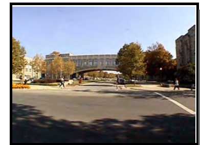
Brick Pedestrian Overpass
