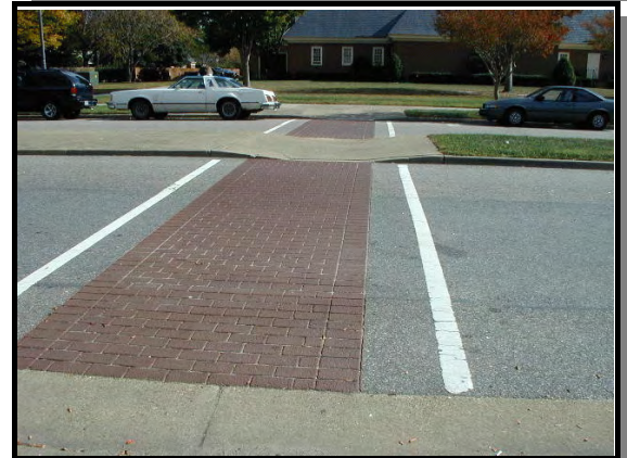
Pedestrian cross walk enhanced by asphalt pavers
