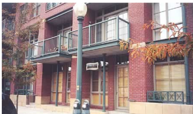
This building makes good use of recessed areas as a means of clearly identifying the entrance
