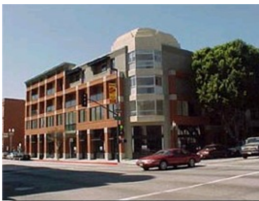
Note the change in material, color, and form used at the corner of this building, clearly designating the entrance
