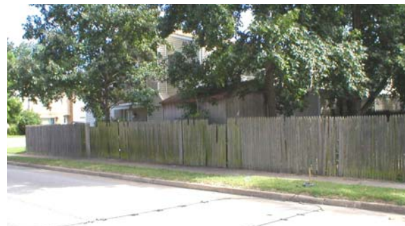
Deteriorating fences along roadway
